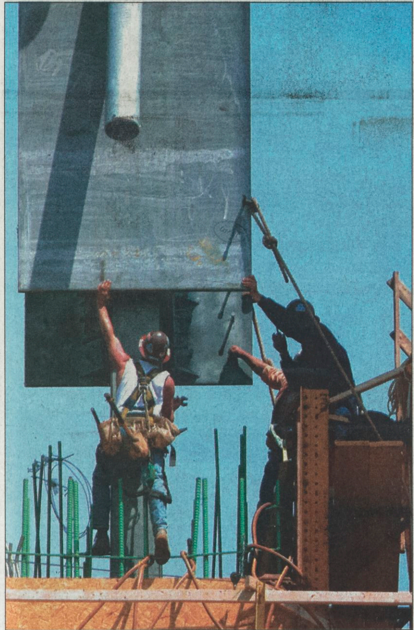
ZACH WITTIG/THE LANTERN Workers help guide one of two tower anchorages into place for the Lane Avenue bridge yesterday. Each anchorage weighs well over 100,000 pounds and required the use of a 550-ton-capacity crane to lift it into place. The project is led by the Franklin County Engineer and prime contractor C.J. Mahan Construction company.
