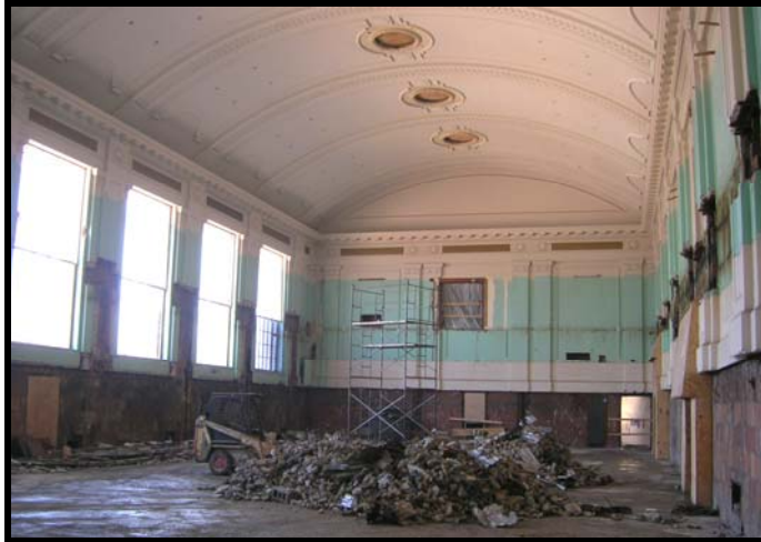
Figure 2: The restored "Grand Reading Room," with the floor dividing it into two floors now removed.
